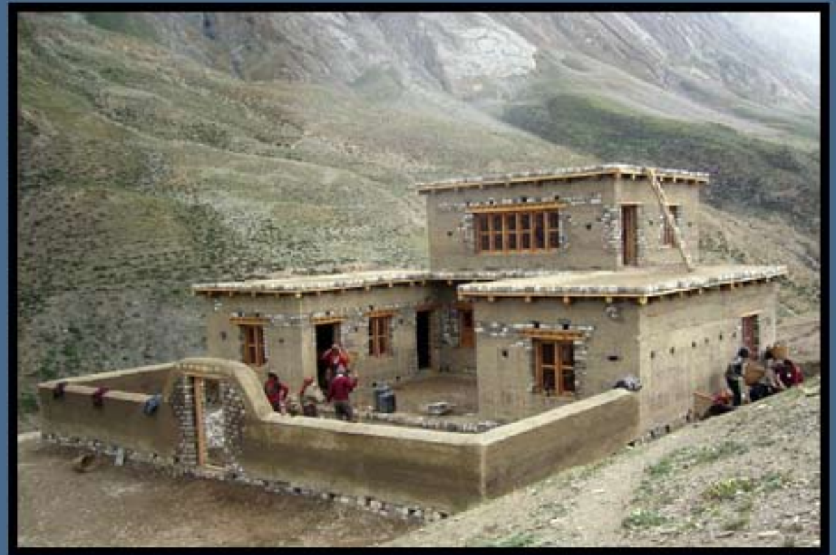
Courtyard walls completed.
