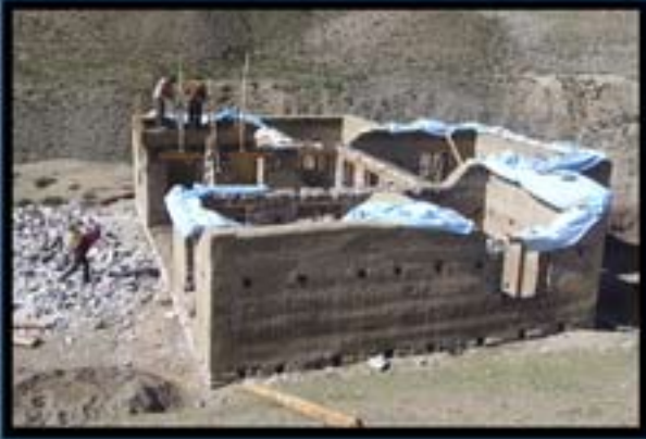
Cement holds rocks and walls together.
