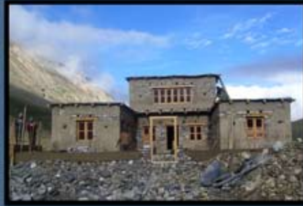
Doorway to courtyard framed, and second floor in place.
